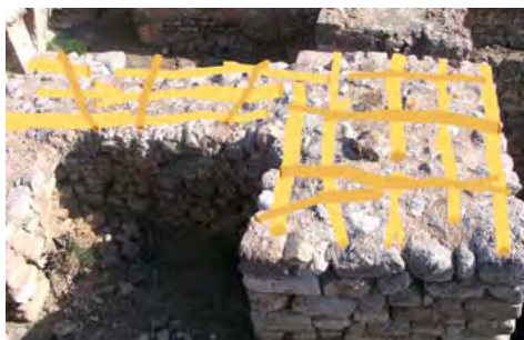
Fig. 8. Phaistos. Grid of horizontal timbers from the first palace as reconstructed by Eleftheria Tsakanika (Tsakanika-Theochari 2009, Fig. 2).
